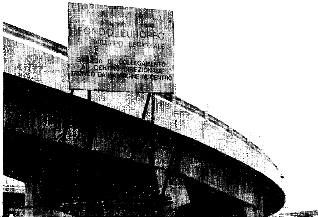
Link roads to serve industrial sites in Naples and Caserta (Italy)
