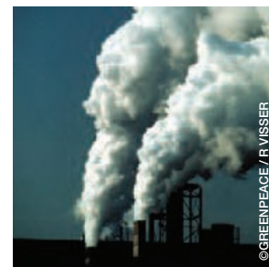
image Blast furnaces of LTV Steel Co, Cleveland, Ohio, USA.
