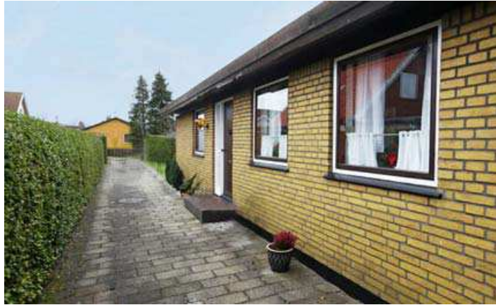
Facade to the North
